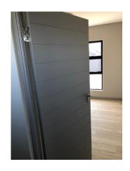
Interior doors: Horizontal slatted hollow core, with 2-lever lock and satin Chrome handles, doors to be painted with eggshell enamel R1450.00 per door including lock and handle.
